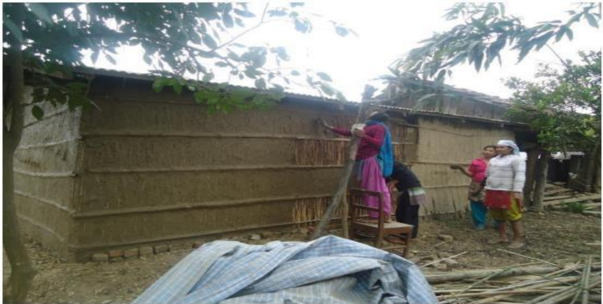
Figure 2-2: Typical Tharu House Building
